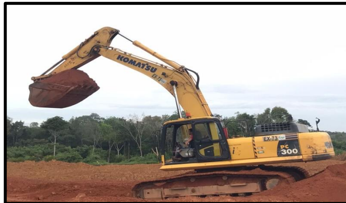
Gambar A.1 Alat Gali Muat Excavator Komatsu PC 300
