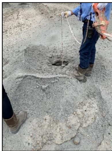
Gambar 4. 4 Sounding Lubang Ledak
