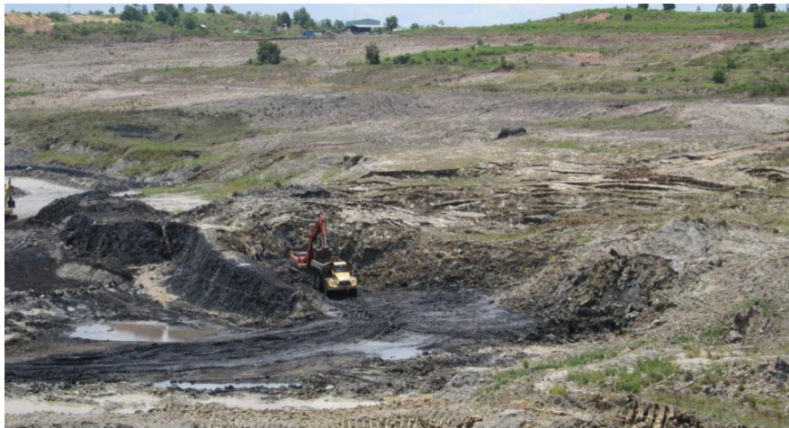
Fig. 8. Excavation using box cut method at low-wall.
