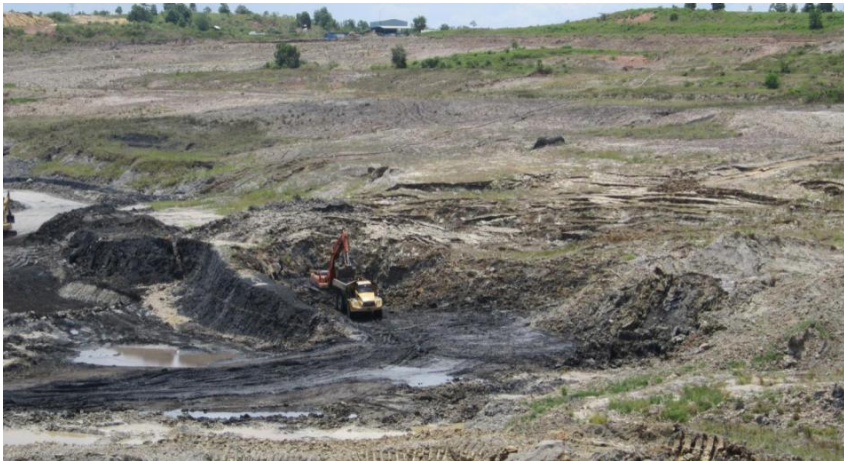
Fig. 8. Excavation using box cut method at low-wall.
