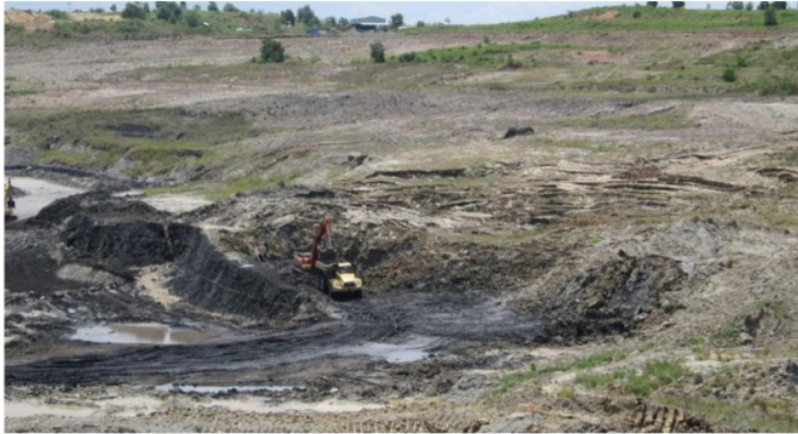
Fig. 8. Excavation using box cut method at low-wall.
