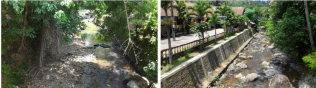
Fig. 9. Deposition on river bed at Loc.1.
