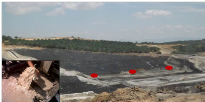
Fig. 14 Depressurization (red dot) and the aquifer stress causing artesian (bottom left)
