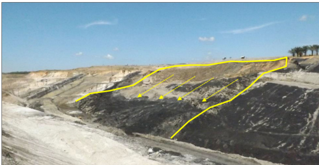
Fig. 8 Failure at low-wall of an open-pit mine
