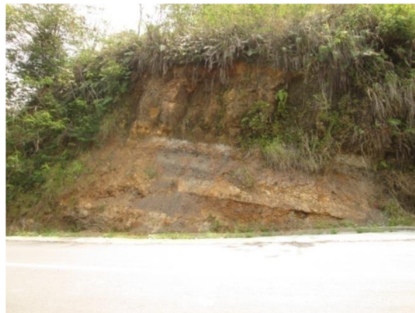
Figure 4. Initial location of MS at KS02B.
