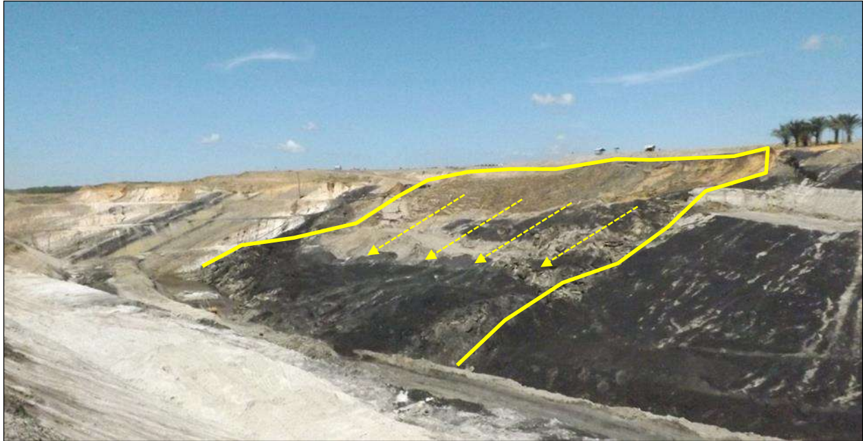
Figure 8. Failure at low-wall of an open-pit mine.
