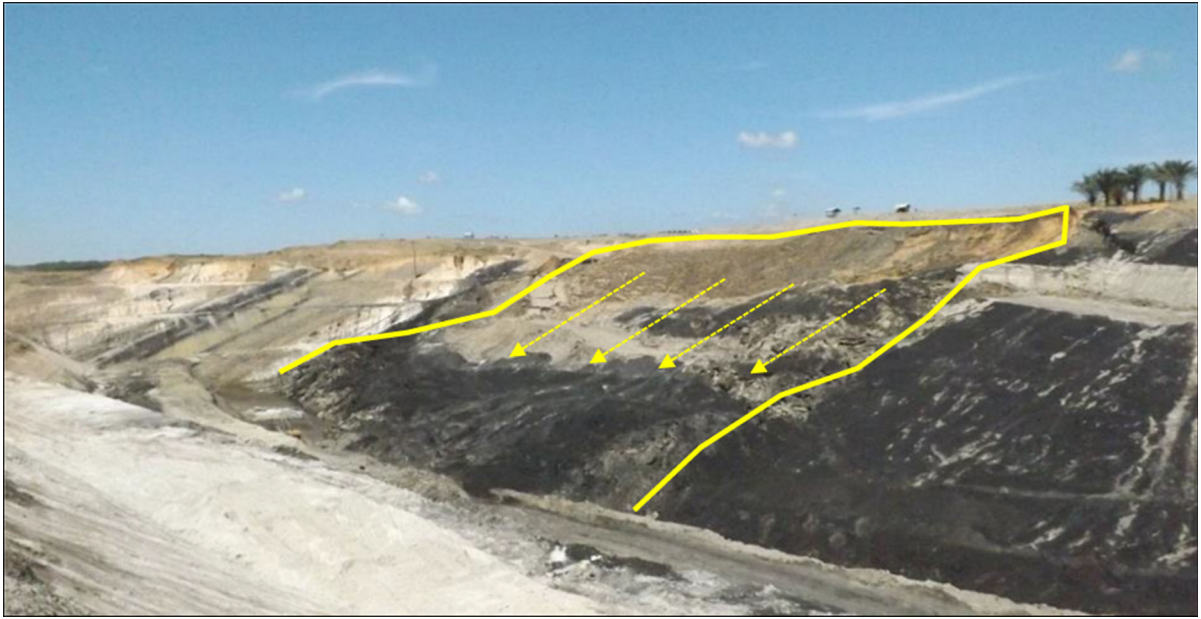
Fig. 8 Failure at low-wall of an open-pit mine
