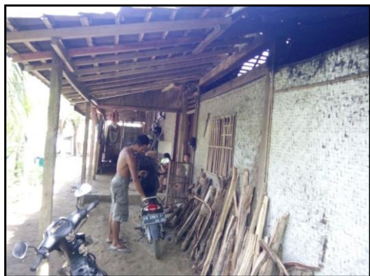
Figure 3. Existing of building
